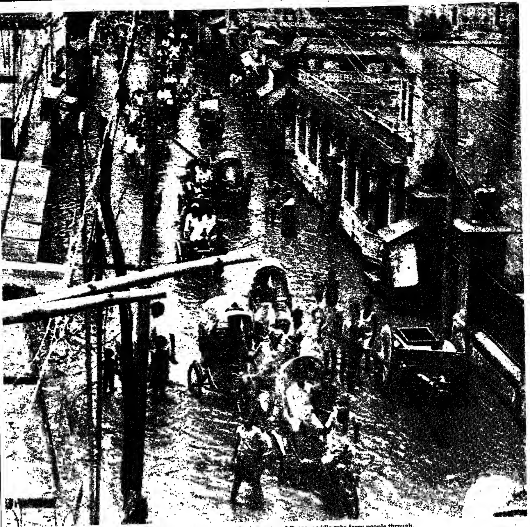
Business as usual: While floodwaters swirl through Kazal Alauddin Street, in the centre of Dacca, peddle-cabs ferry people through.
